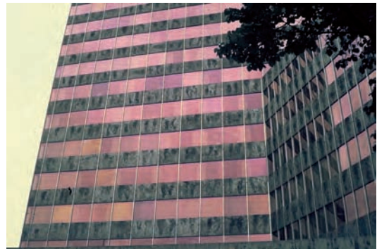
Figure 1.17 First efforts to overcome the effect of large areas was to reduce the transmission of glass by reflective and absorptive glasses
