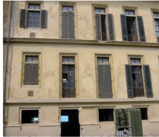
Figure 13.4 Refurbished traditional louvre shutters on south elevation
