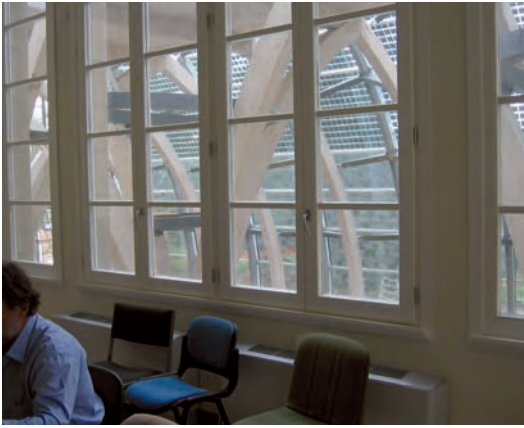
Figure 13.3 Replacement timber windows with low-e glazing
