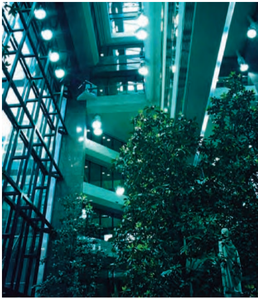
Figure 6.11 This exotically planted atrium required permanent artificial lighting due to the choice of green glass for the envelope
