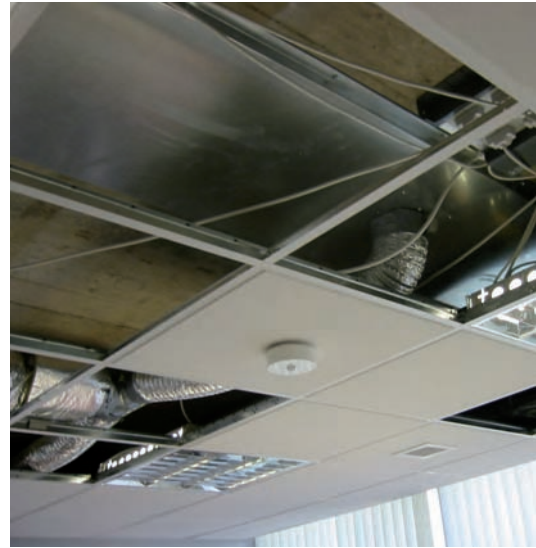
Figure 11.4 The CoolDeck system: Air is drawn between the concrete slab and metal trays containing PCM
