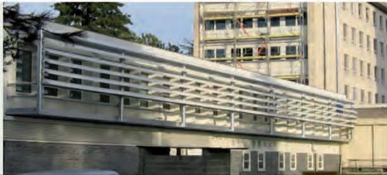
► Figure 12 Fixed external louvres may improve light uniformity but interfere with view out
