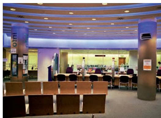
Figure 11.9 The LED lighting system in the Customer Service Area is of high luminous efficacy and is programmed to make changes in colour to add visual interest to the waiting area
