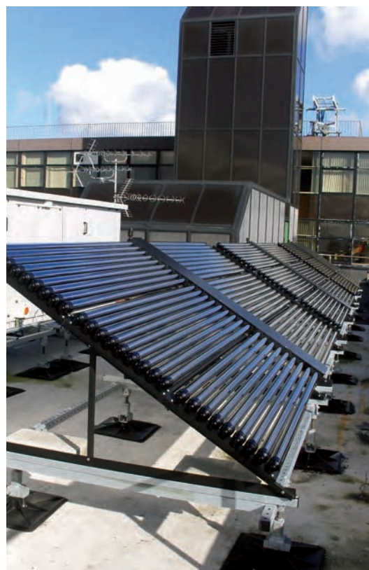
Figure 11.10 The evacuated tube array of solar thermal collectors contributing to domestic hot water
